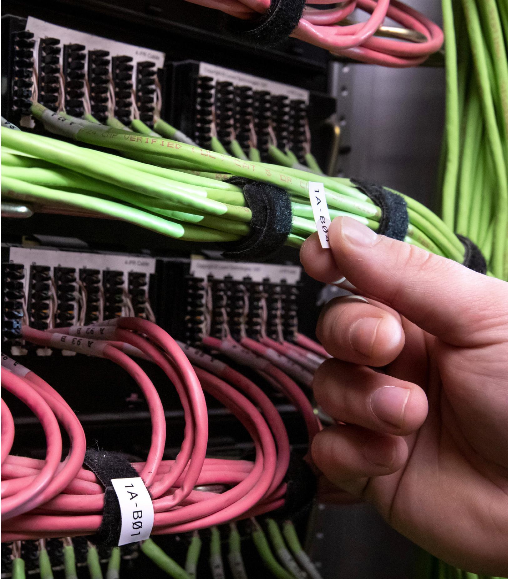
Label printed on the BMP®41 Label Printer using B-414 BradyGrip™ Print-on Hook Material (MC-500-414)
