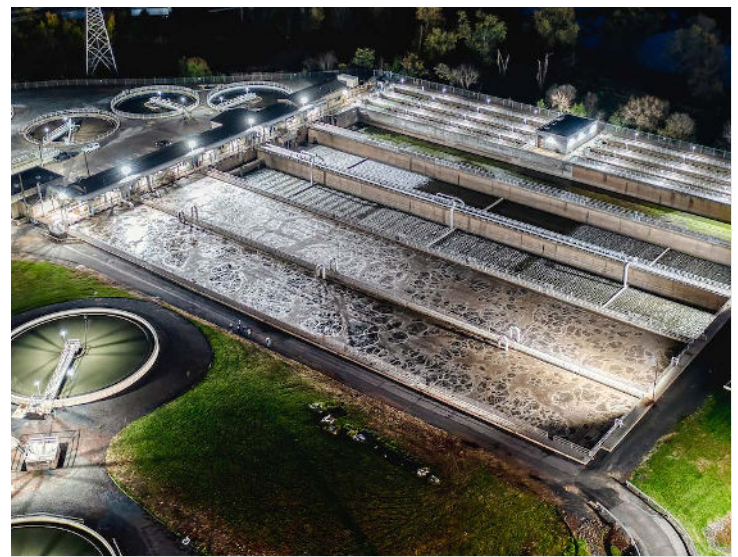
Dialight LED fixtures illuminate the exterior tanks in Bridgewater, NJ.
