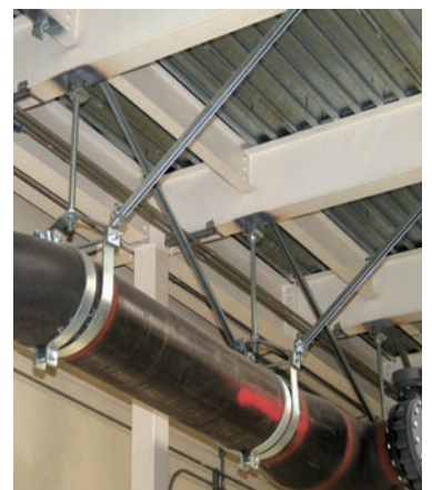
TOLCO seismic bracing
