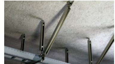
TOLCO seismic bracing
