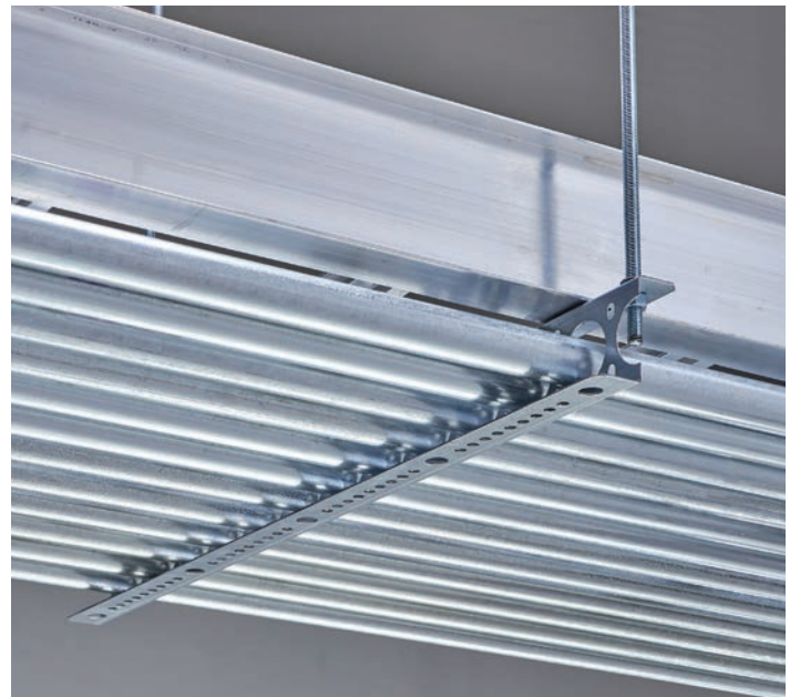
Conduit trapeze support with cable tray
