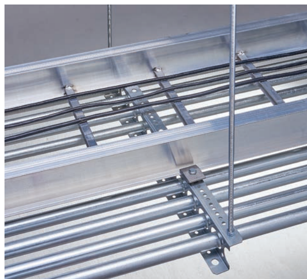
Conduit and cable tray trapeze support
