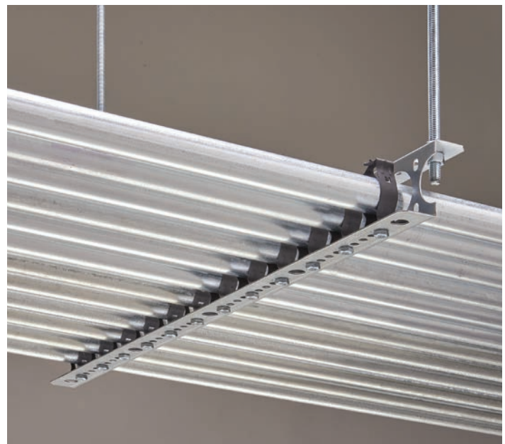
Conduit trapeze support with Guide-Rite™ fasteners
